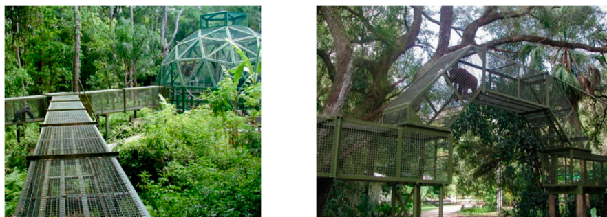
Figure 6. Elevated animal rotation raceways or "trails" developed at the Center for Great Apes in Wauchula, Florida (Photos: Center for Great Apes).
